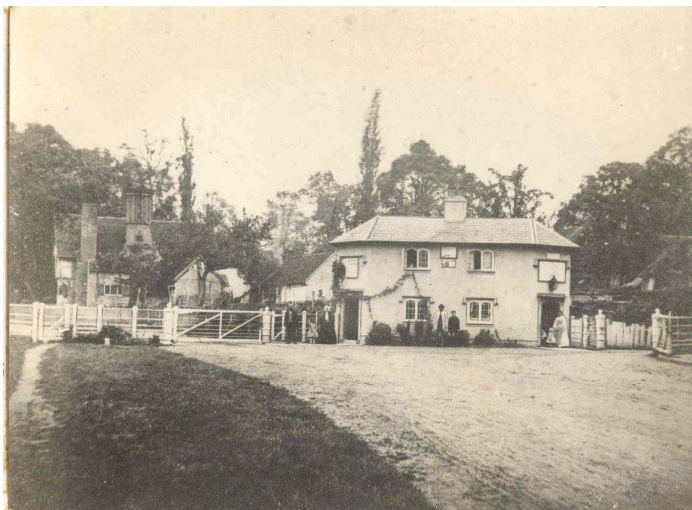
The Arrow toll-house showing very similar gate posts to those standing outside Beauchamp Court. No doubt the turnpike trust acquired the posts for all the toll gates from the same supplier. These two gates blocked the Evesham road and the Worcester road. The toll-house has managed to survive to the present day.
