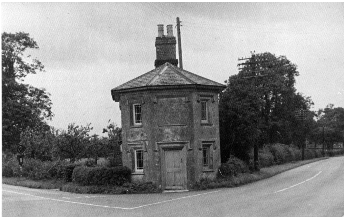
The toll-house that stood on Birmingham Road was erected in 1839 (known in the Trust's minutes as the Alcester Turnpike House) and was demolished in 1950s.
