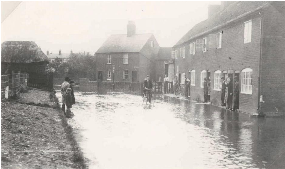
Floods in School Road, Alcester c1950 [ADLHS Archive]
